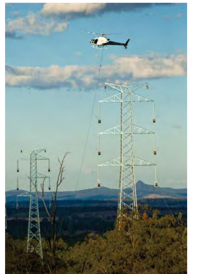
Helicopter stringing of conductor over forest canopy
