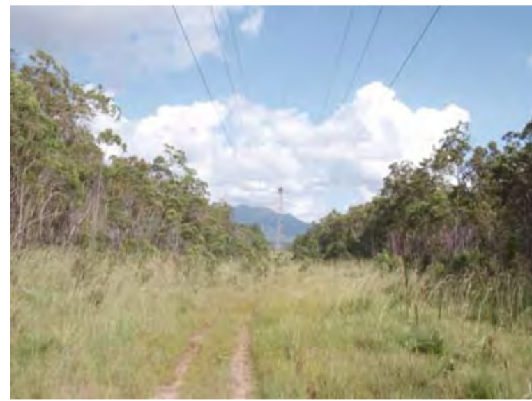
Powerline easement showing sculpted easement clearing
