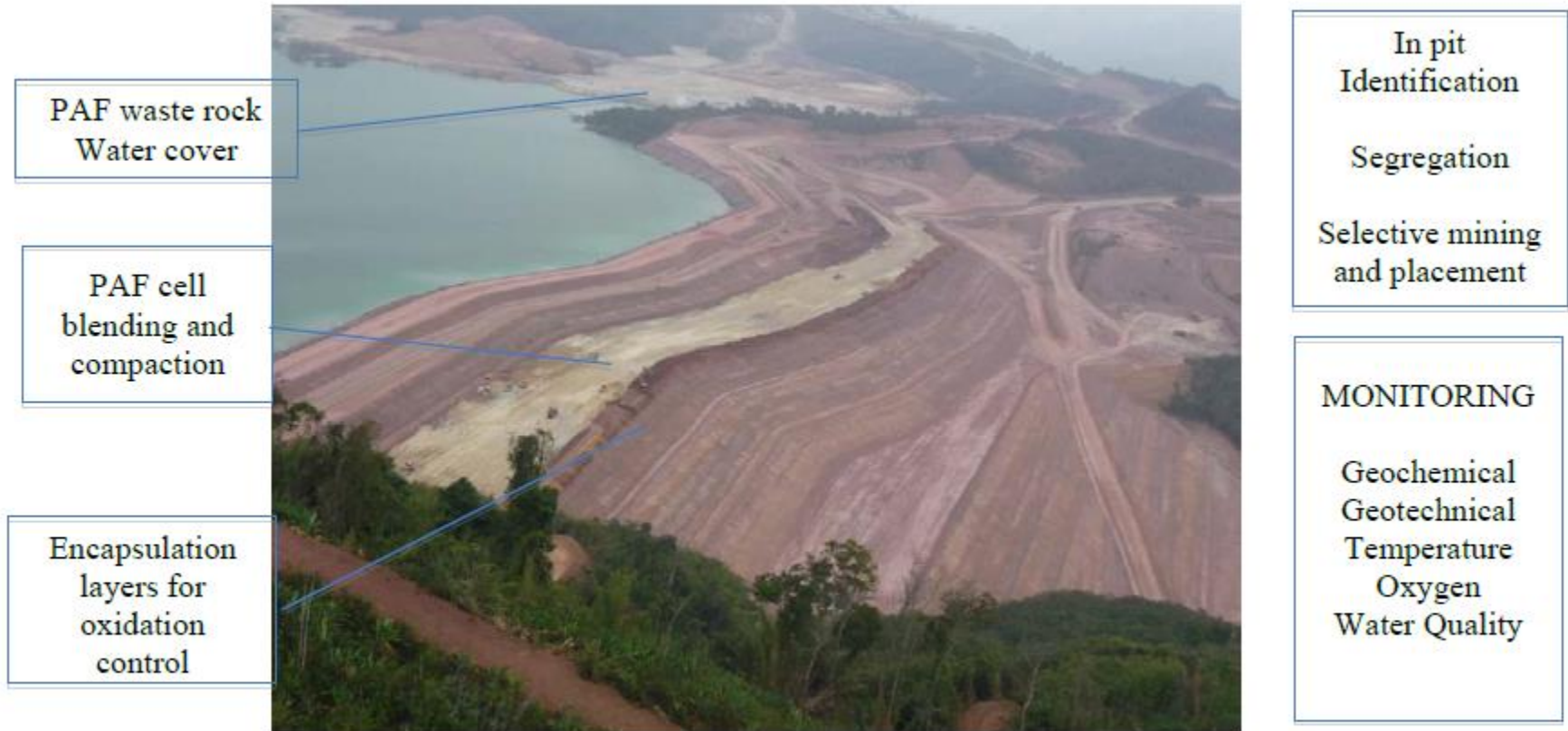
Fig. 6. Waste Rock Management for ARD Control at the Phu Kham Mine in PDR Lao
