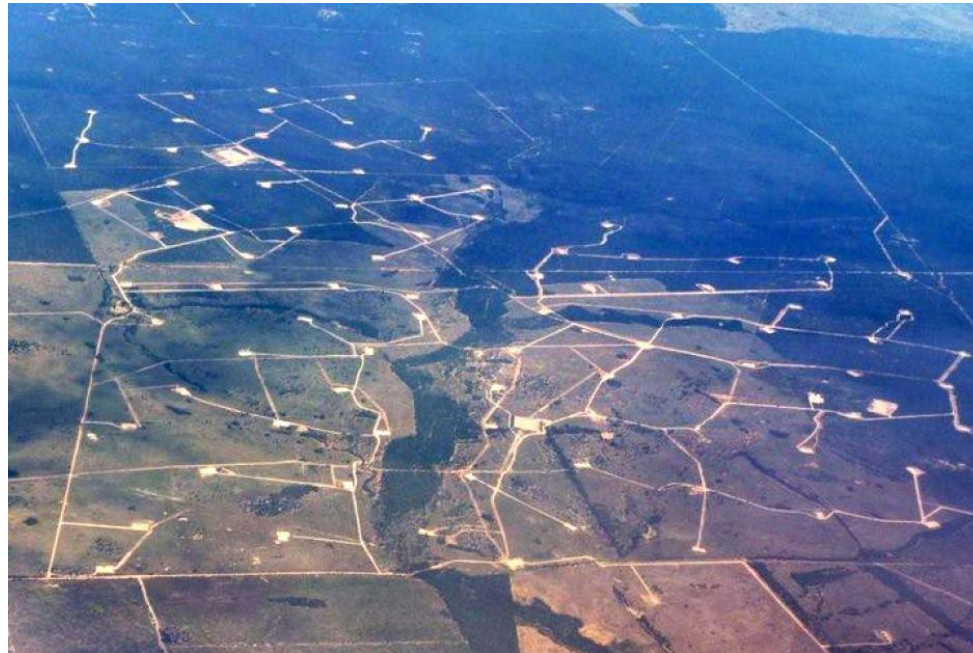
CSG gas field (~2012)
