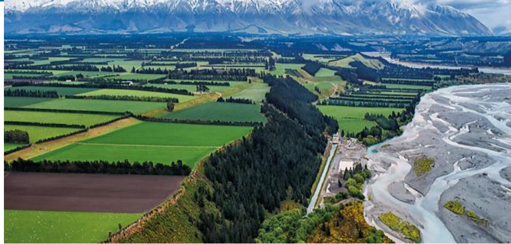
Highbank power station on RDR tail race
