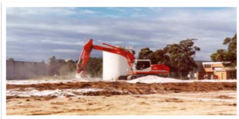
Lime enrichment and composting degrades hydrocarbons
