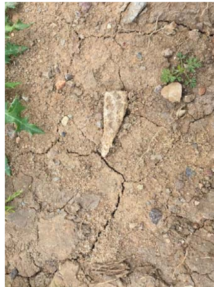
Suspected Asbestos after a residential site had been remediated
