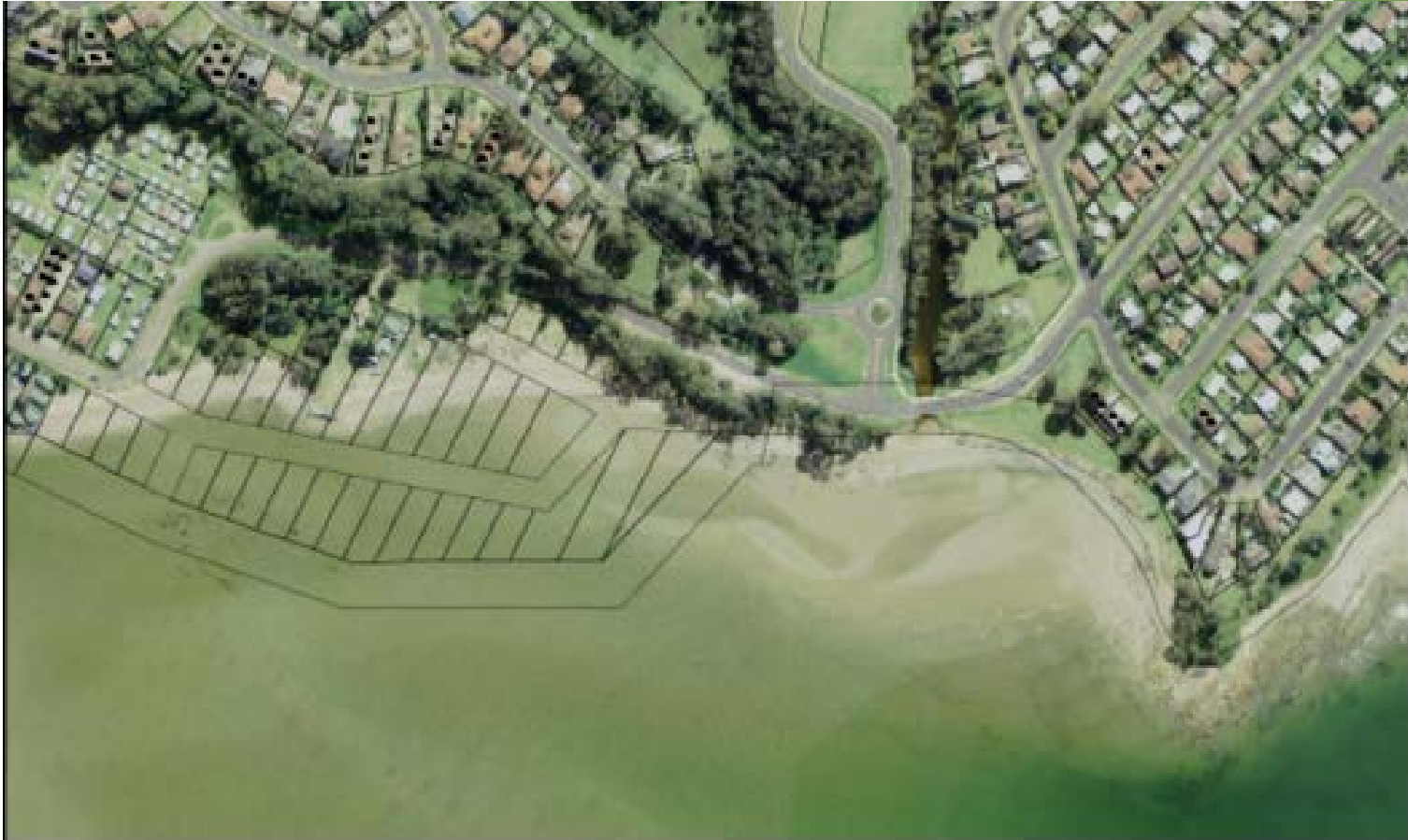
Shoreline recession at a coastal erosion hotspot, courtesy of Eurobodalla Shire Council.
