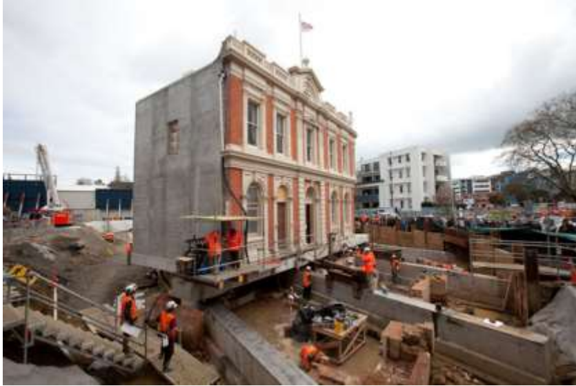
Victoria Park Tunnel, Auckland
