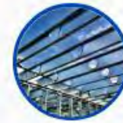
Suspended steel structure
