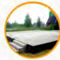
Concrete slab on ground
