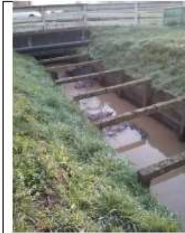
A fish screen that was blown out in a storm. Area had to be re-fished.
