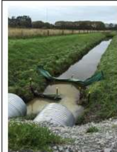
Silt fence used as a fish screen. Is this idea?
