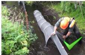
The fish screen has been overtopped and fish can get in between gaps in the steel plates. This site needs to be reassessed, and possibly fished again.
