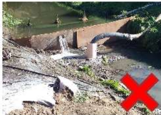
The fish screen has been overtopped and fish can get in between gaps in the steel plates. This site needs to be reassessed, and possibly fished again.
