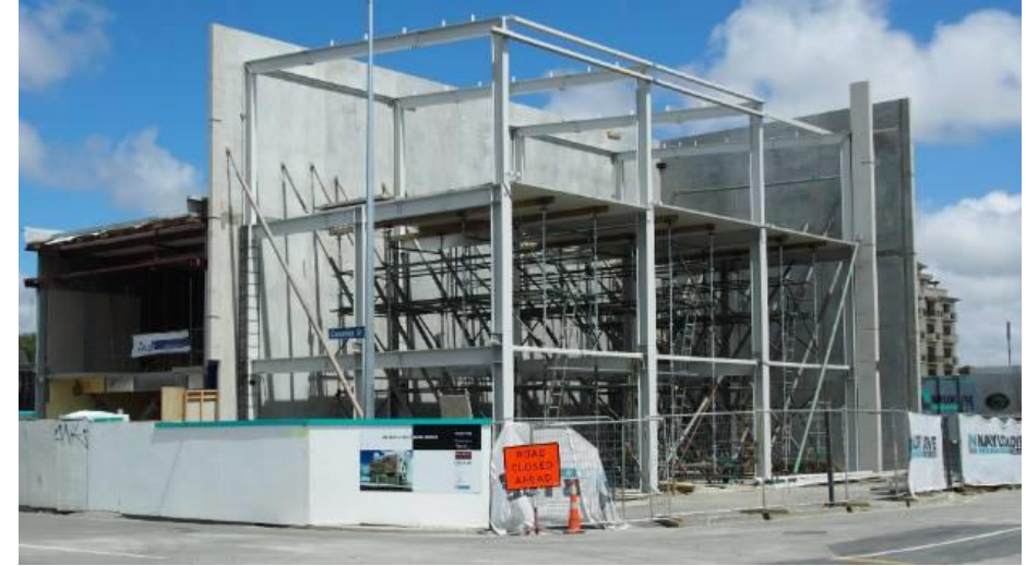
Typical steel frame construction with reinforced concrete slab walls in Christchurch
