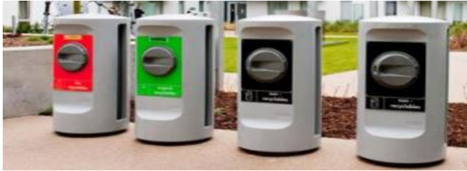
Wembley Envac Residential Waste Inlets
